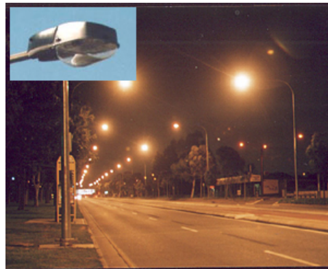
Source: www.astro.caltech.edu/.../images/viewjian2006 : Bad example of public lighting
